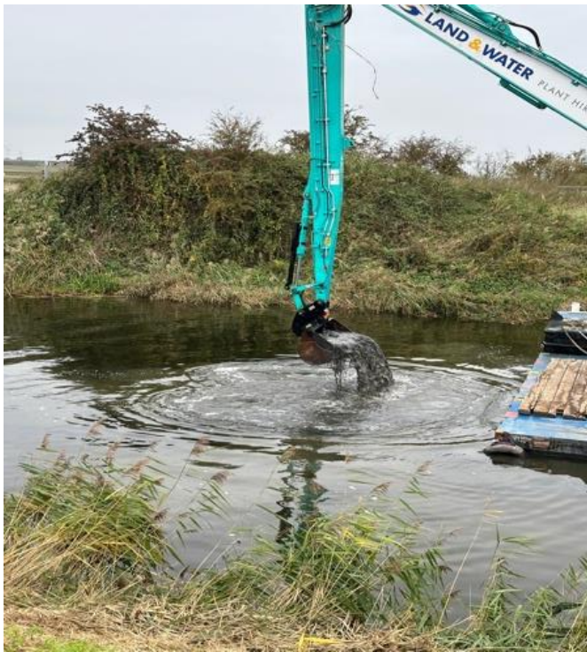
The first bucket lifted at Cottons Corner
