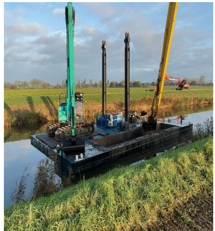
Machinery used for lifting silt onto the embankment
