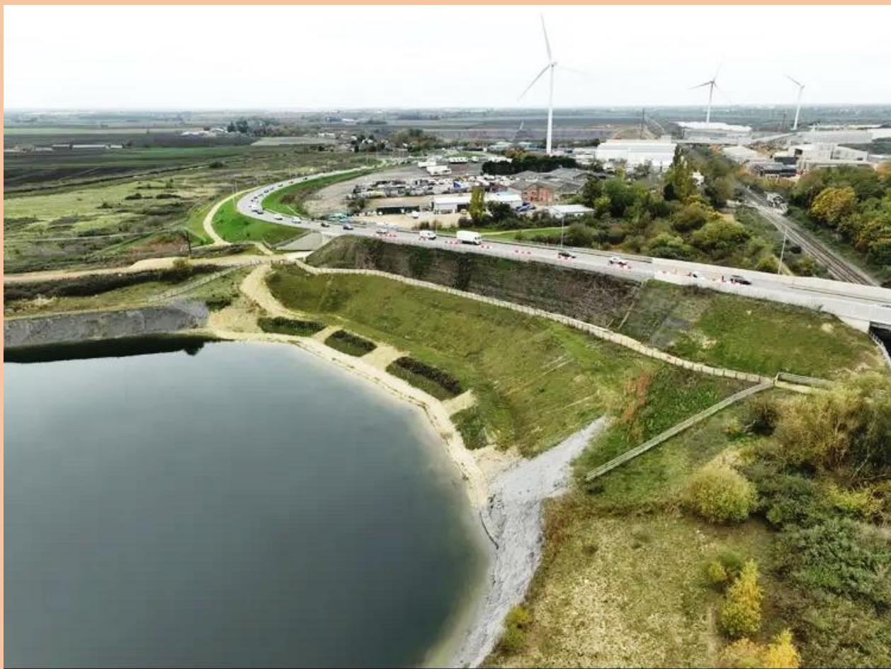
Picture shows how 'steep' the support embankment is.
