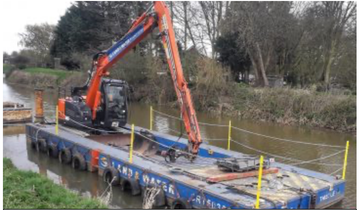
Pontoon and excavator similar to what we will use
