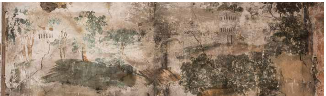
Fig. 44. Paint loss is widespread and can be attributed to a number of different damage and deterioration mechanisms.
