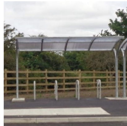
Figure 3 - Manea Railway Station Cycle Parking
