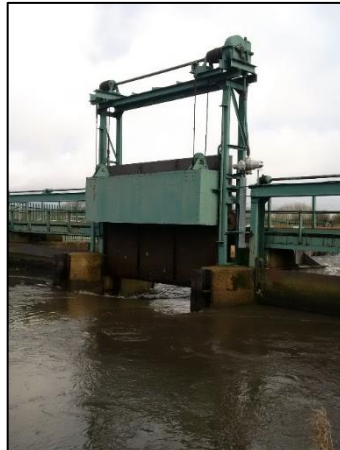
Stanground Sluice in operation
