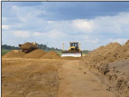
2012-15 South Barrier Banks Scheme
