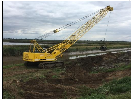
De-silting of the tidal River Nene, on behalf of the EA, by North Level District IDB
