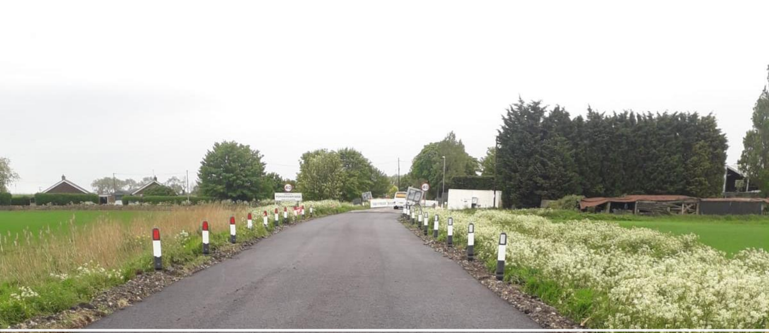
Section 1 Bollard Installation Works – Ramsey Road
