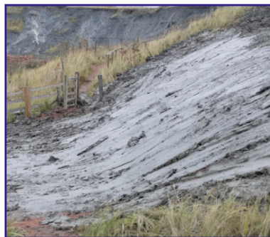
Re-cut slope © Copyright Philip Parker
