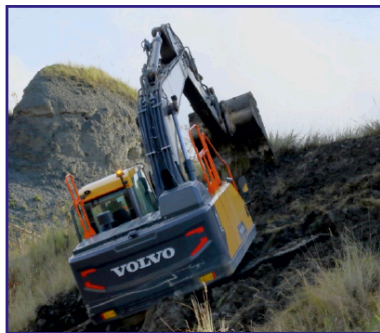
Clay slippage being reprofiled © Copyright Terry McKenna
