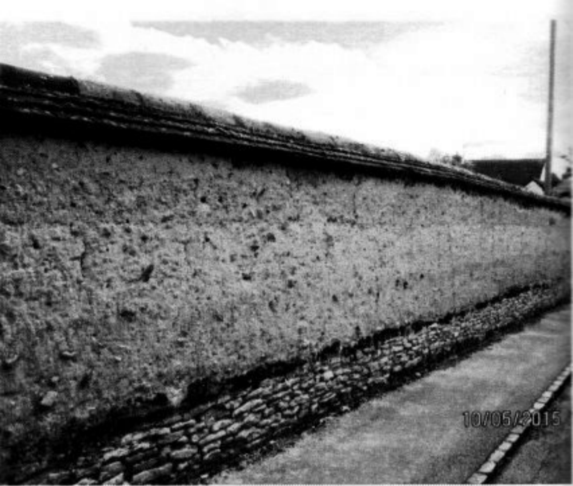
Typical Mud wall
