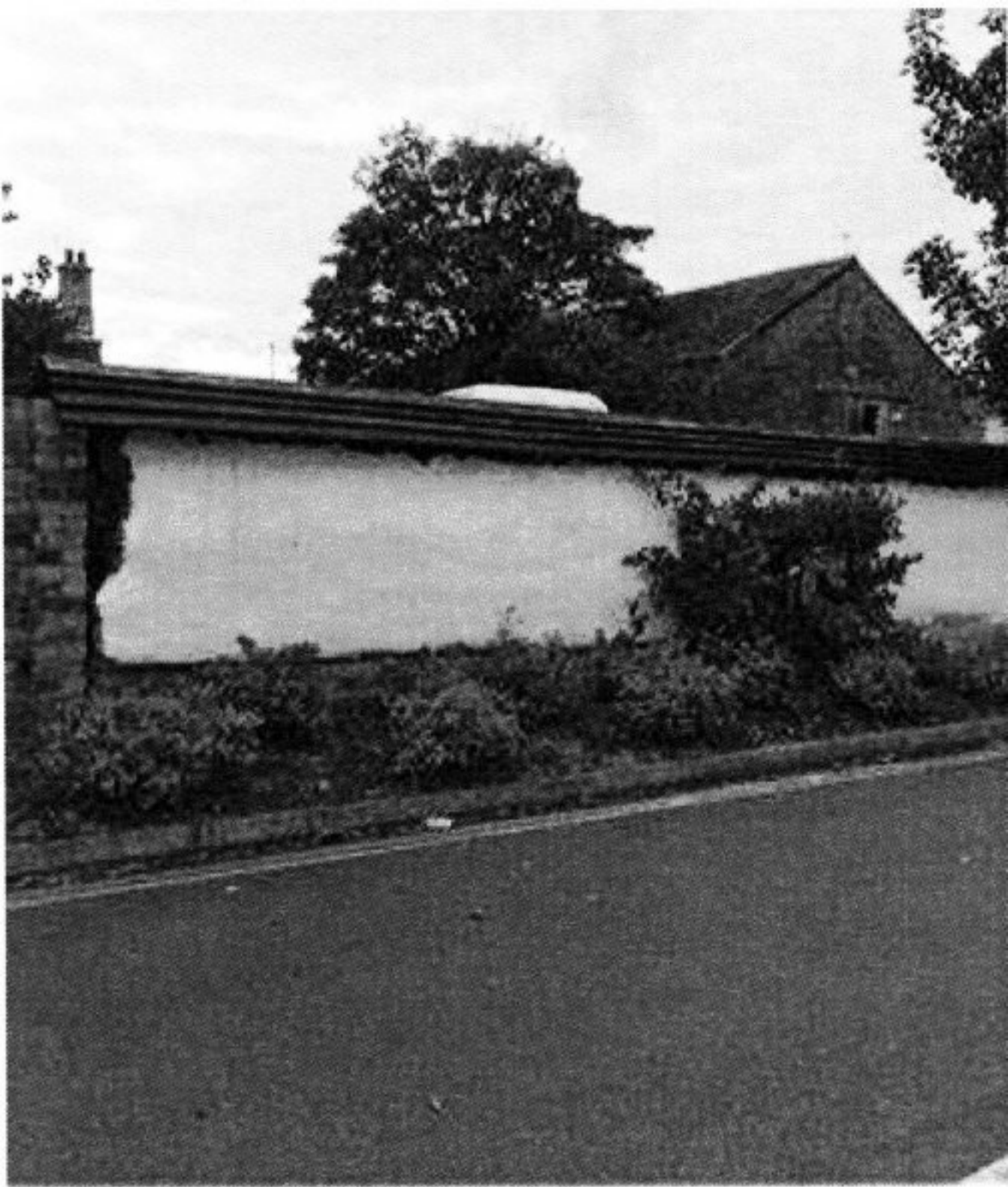
Mud wall with tiled coping
